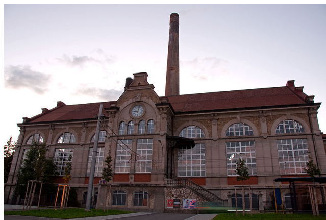
Exhibit 2 - Power plant built in 1906 in La Chaux-de-Fonds, now protected by UNESCO (image source: http://en.wikipedia.org/wiki/File:UsineElectriqueLaChauxDeFondsCH1.jpg )
